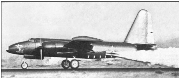
The Neptune during a 14 second JATO burn on takeoff.
